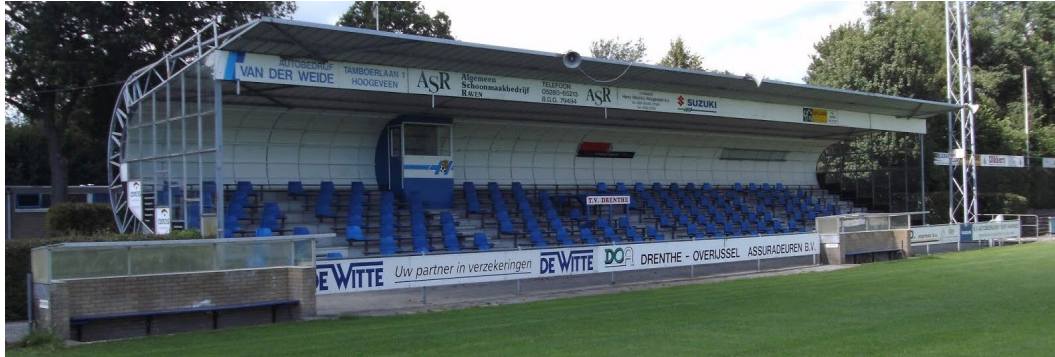
Left The original Elascan stand served the Hoogevens club since its construction in 1976
