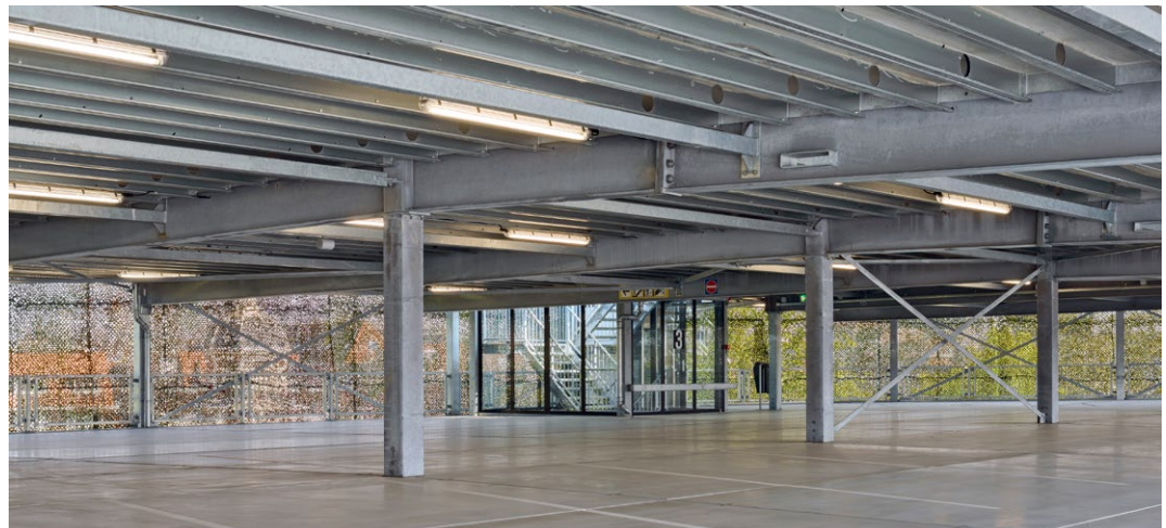
Left and right This car park at Moorsport in Leiden was designed in galvanized steel to ensure it can be easily dismantled and relocated
